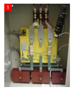
a clamping voltage of 267 volts. The actual clamping voltages are shown in photographs 2, 3, & 4 (page 2). When you consider that you do not want to begin to clamp an impulse at less than 120% above nominal, (144 volts), and that a typical 120 volt rated TVSS' unit utilizes 150 volt MOVs, a clamping voltage of 187 volts is extraordinary. The difference in clamping voltage between the technologies is 80 volts, or an improvement of 316%, over an MOV only system.
